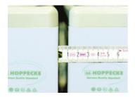
Fig. 5-14: 10 mm clearance between the batteries
